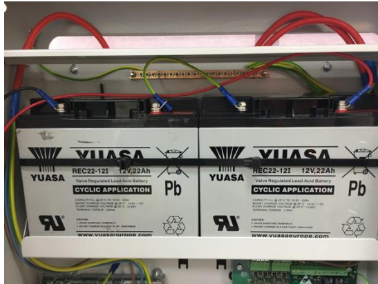
PHOTOS 1 & 2 SHOWING LOCATION OF BATTERIES AND CONNECTIONS TO THE POWER SUPPLY PCB
