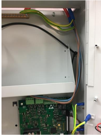
PHOTOS 1 & 2 SHOWING LOOP CABLES ROUTED AND CONNECTED TO THE MAIN PCB
