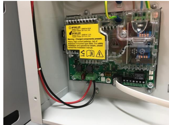
PHOTOS 1 & 2 SHOWING LOCATION OF BATTERIES AND CONNECTIONS TO THE POWER SUPPLY PCB
